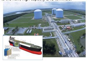
Figure 8: LNG terminal at Bba Island/ GA. The inset schematic of an LNG super tanker exhibits a hull with multiple shells. On the left a multi-layered super insulating double-hull cutout. After (DOE-NETL, 2005)
